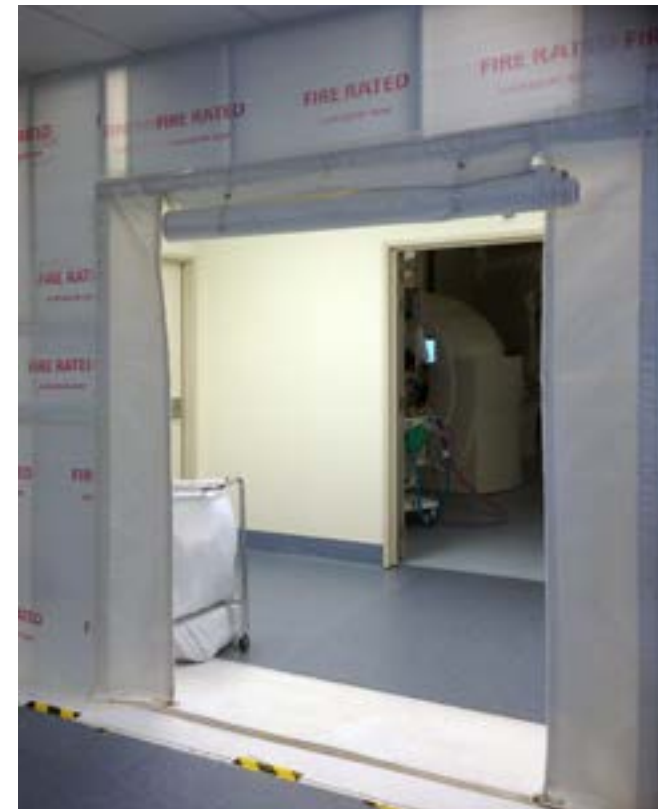
Corflute barriers and heavy-duty zip seal doors allow scanning and procedure rooms for all patients being managed under droplet or airborne precautions to be sealed off.
